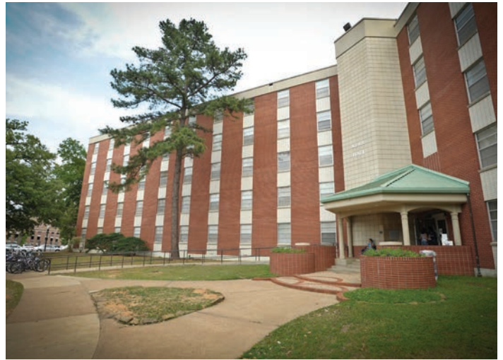
KERR HALL: Female / Shared Room / Community Bathroom
